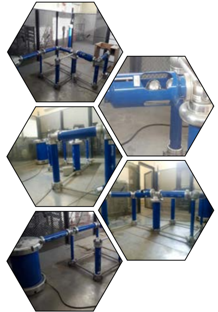
High Voltage Laboratory.
