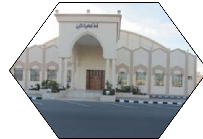
Auditorium with approximately 300 audience seating capacity.
