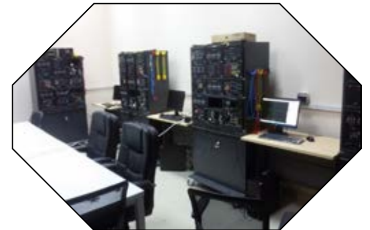
Power Electronics Laboratory.
