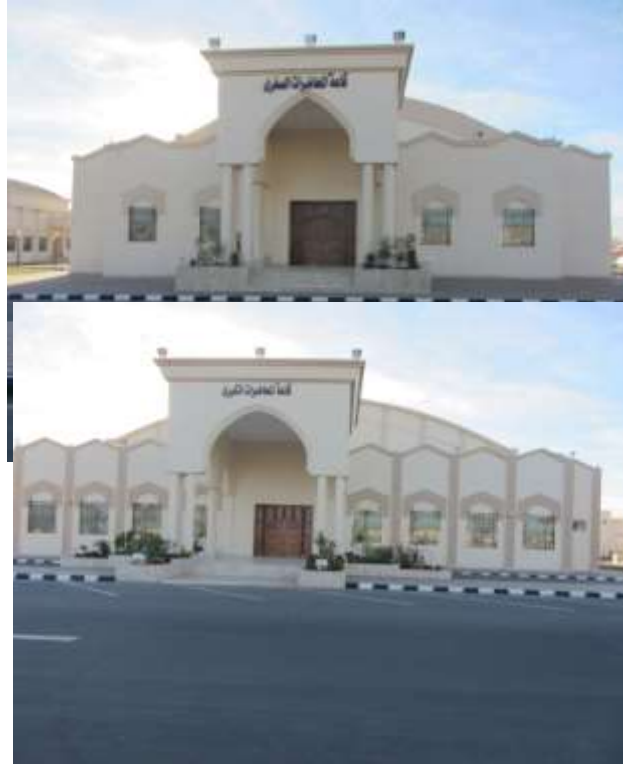
Auditoria Hall with Approximately 300 Seats
